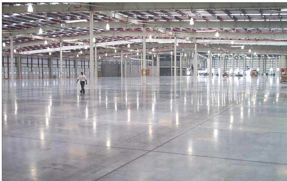
Wal-Mart facility, Guadalajara, Mexico
